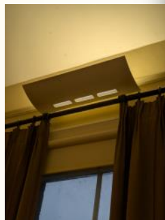
The uplighters in the main hall
